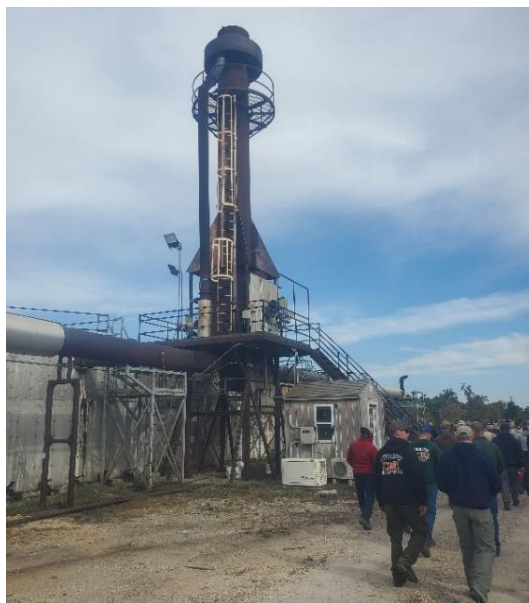
Kilns are connected to an incinerator that burns smoke and other byproducts and reduces emissions. Photo credit: Chris Lohmann.
